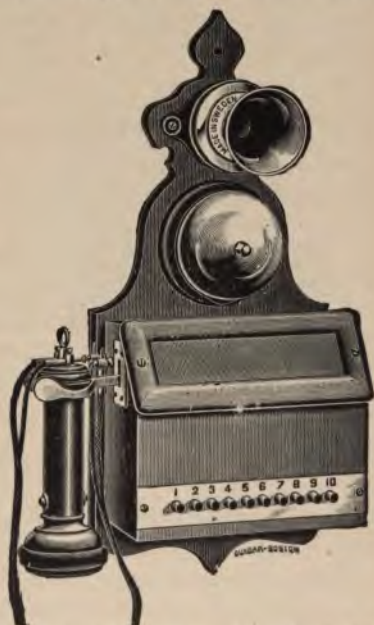
FIG. 206.—Station apparatus equipped with a ten-point Plummer switch.
